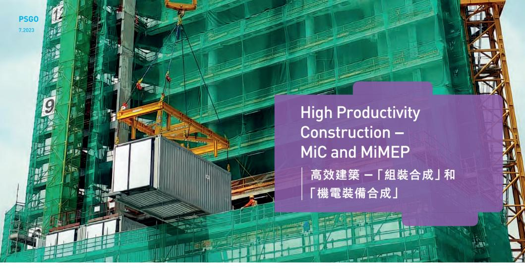
PSGO is actively supporting High Productivity Construction (HPC) methods such as Modular Integrated Construction (MiC) and Multi-trade Integrated MEP (MiMEP) to tackle the challenges faced by the construction industry. HPC enables labour intensive construction activities to be transferred to the factory, so as to reduce on-site labour, thus uplifting the on-site productivity and enhancing performance on works quality, site safety and environmental sustainability.
